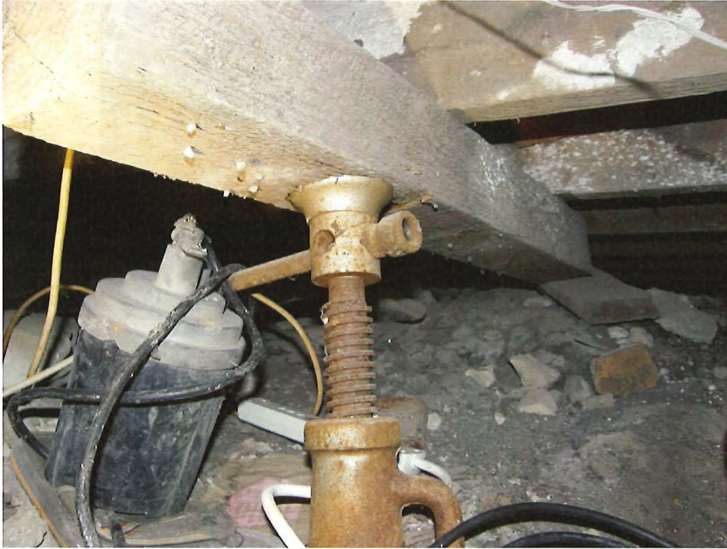
Jack added to stop floor from falling
