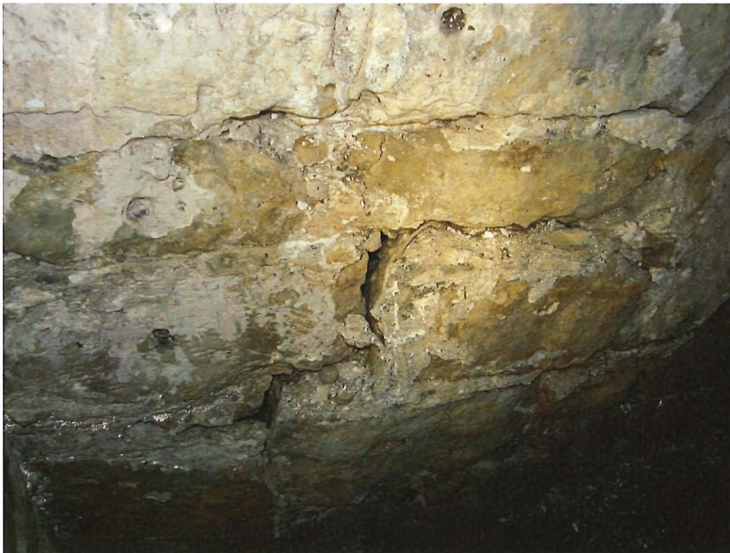
Foundation Cracks
