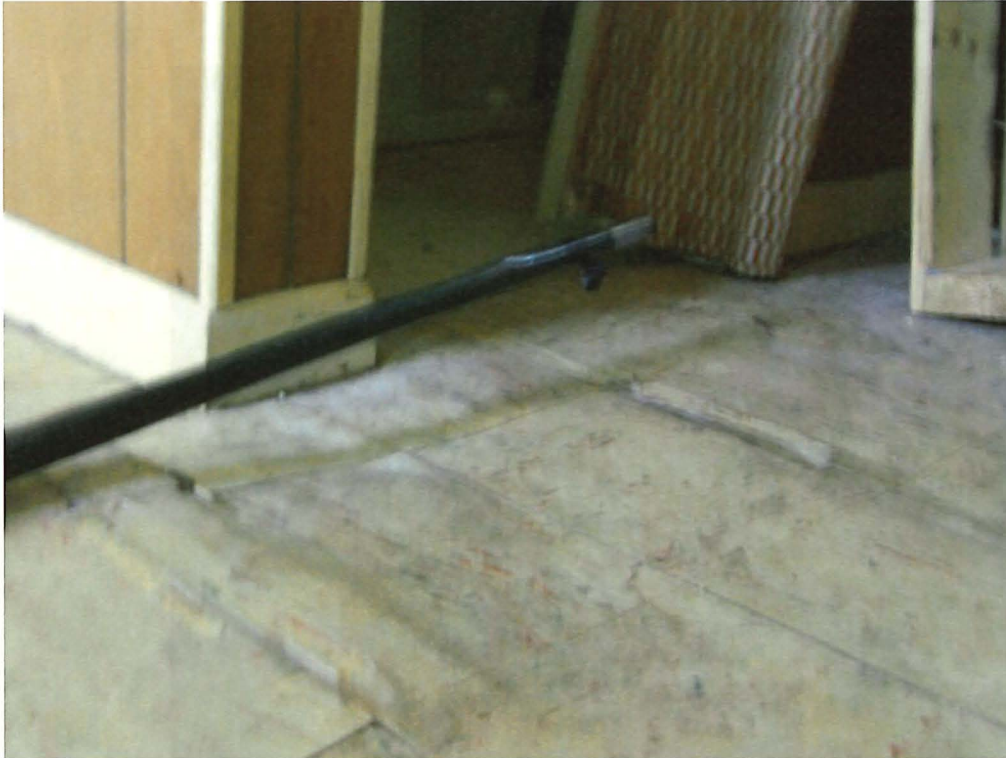
4" out of level in a 2' area
