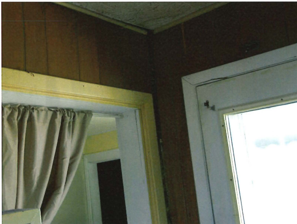
Inside picture of addition wall pulling away
