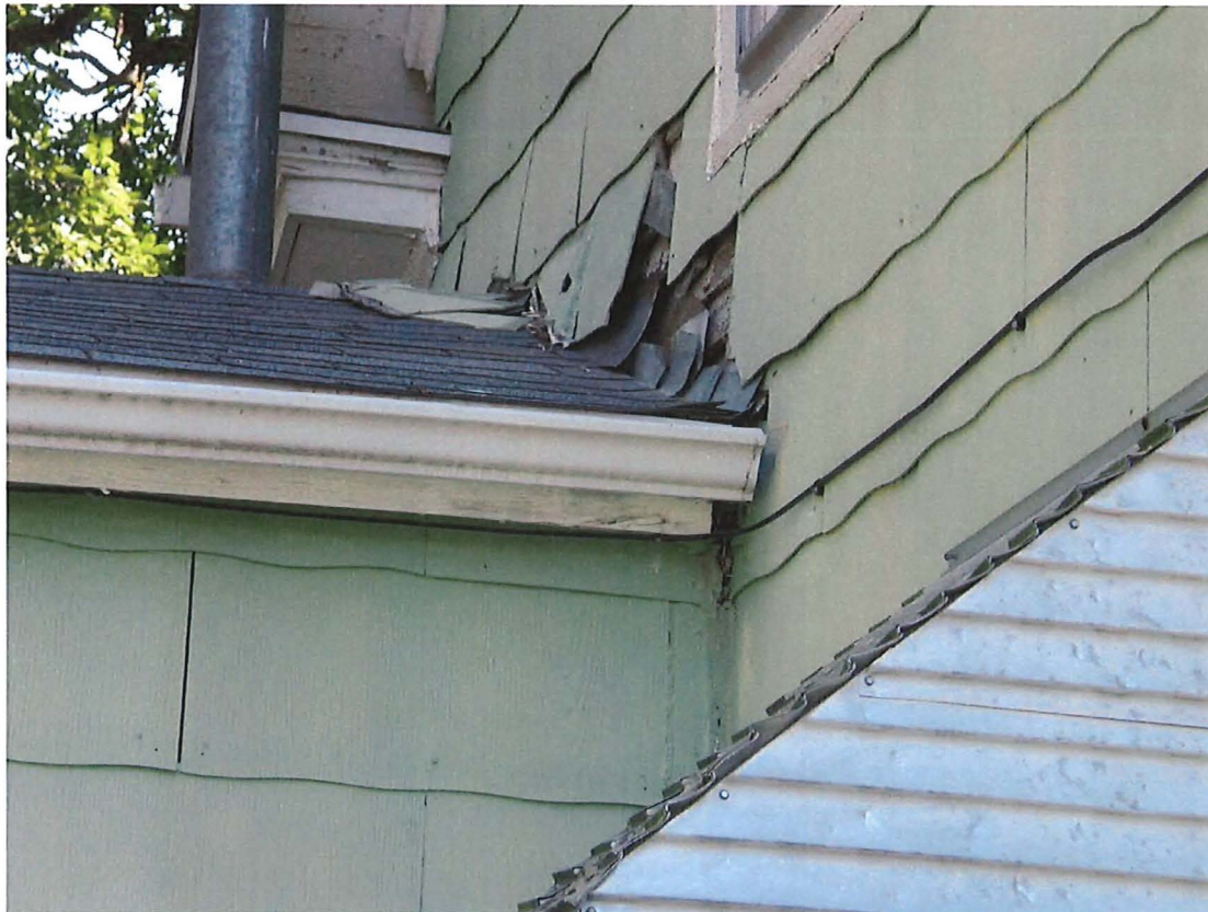
Outside picture of addition pulling away.
