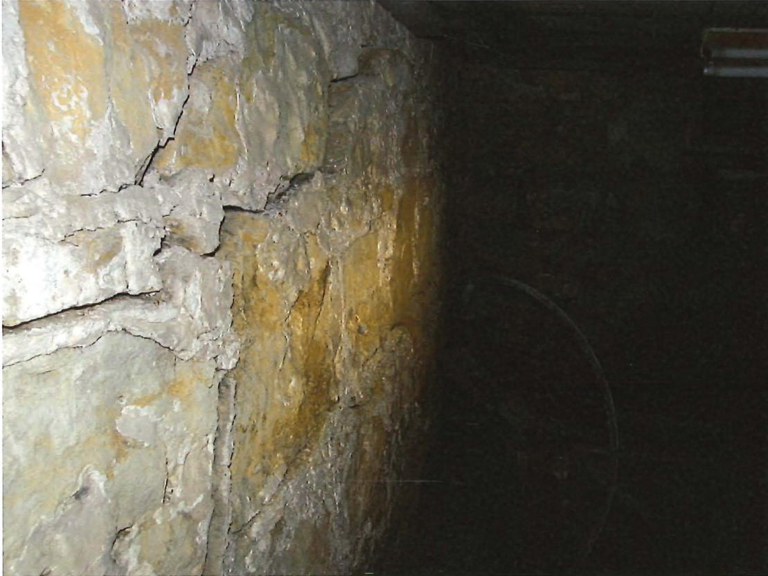
Foundation Cracks
